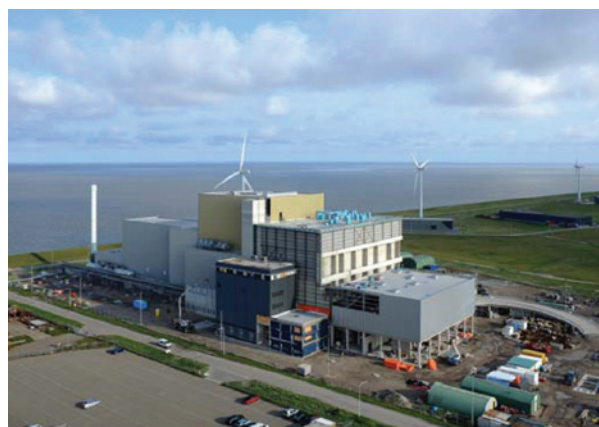
OMRIN - REC Harlingen Waste-to-Energy 1x28 t/h
