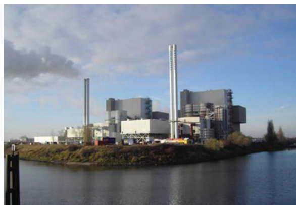
MHKW Magdeburg-Rothensee Waste-to-Energy 4x22 t/h
