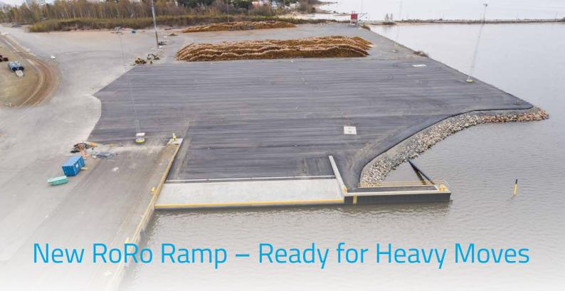
Completed in 2024, the new RoRo ramp at Kallonlahti in Mäntyluoto Harbour introduces a new mode of cargo handling at Port of Pori, serving the needs of industry, project logistics, and defence transport. With a draft of 10 metres, the ramp can accommodate larger vessels safely and efficiently. The ramp itself measures 40.5 metres in length, providing ample space for the loading and unloading of heavy and oversized cargo.
