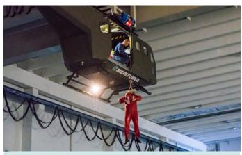
The safe pool environment enables effective training year-round and in all weather conditions. The winching helicopter simulator accurately replicates a real evacuation scenario.
